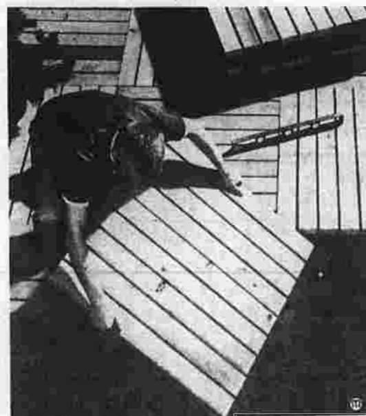
USE PRE-ASSEMBLED SECTIONS atop well-prepared earth surface to assemble deck. One of many dollar-saving tips from new book, Improving the Outside of Your Home, from Structures Publishing Company.
