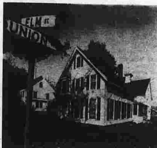
PRE-FINISHED ALUMINUM SIDING restored this old colonial-style house to its original beauty, and aluminum trim preserved special architectural details around windows and doors. Insulation installed behind the panels helps reduce fuel use. With warranties of up to 40 years, aluminum siding more than repays its original cost by eliminating need for repainting.
